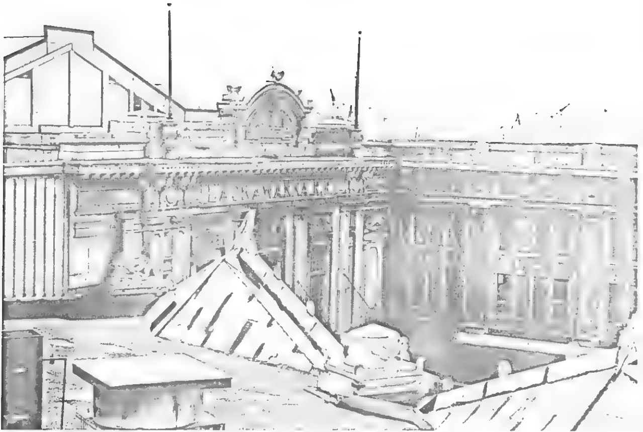
View from the roof of the ferry building, looking southwest toward northern facade of waiting room.
